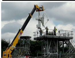
Installation of new direct broadcast reception system at Exeter in 2024. Photo: Nigel Atkinson.
